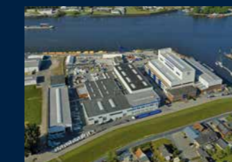
Fassmer Headquarters Germany | Berne
